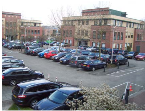
Figure 5.1: The Logica building, located in Rotterdam
